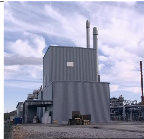
Figure 31 Gas-to-Liquid, Tjelbergodden Plant in Norway, commissioned in 1997. Capacity 1000 mill. liters per year
