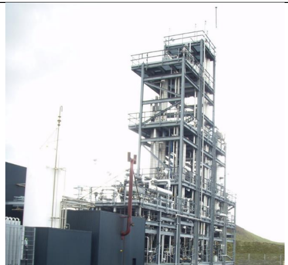
Figure 32 Power-to-Liquid, George Olah Plant in Svartsengi, near Grindavik, Iceland, 2012. Capacity 5 mio. liters per year.
